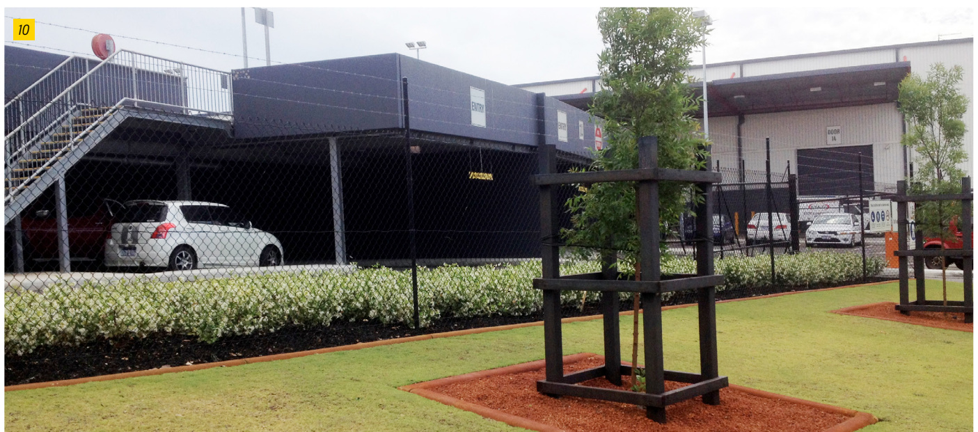
Figure 10: Decked Parking At The Stockyards Industrial Estate
