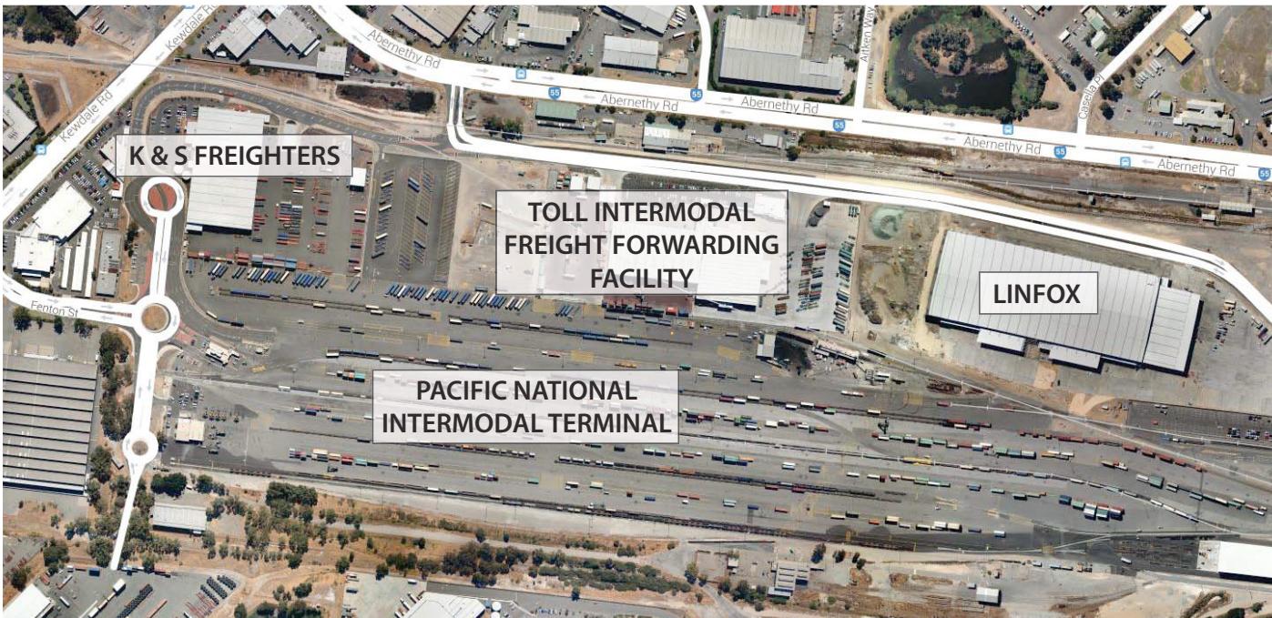
Figure 2: Aerial of The Perth Freight Terminal
